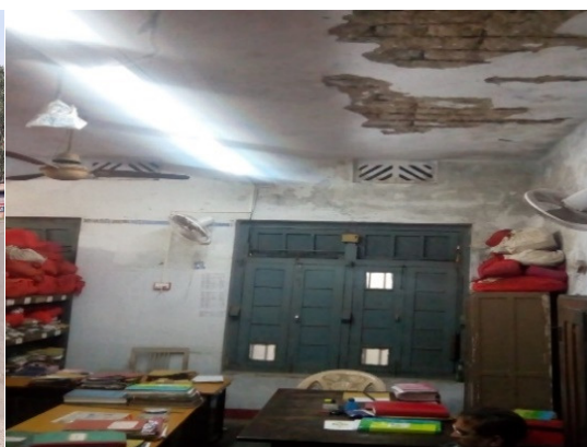
Room with damaged ceiling being used as Reserve Office at East Singhbhum PL (23/10/2018).
