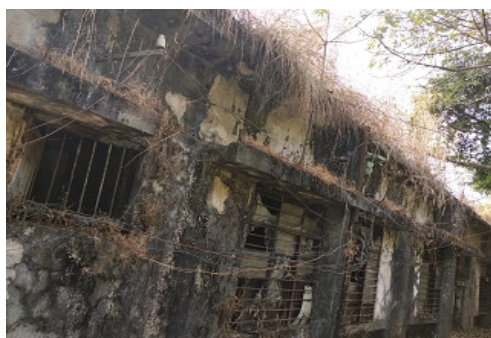
Building of Sadar PS, Ranchi which needs immediate repair (20/12/2018).
